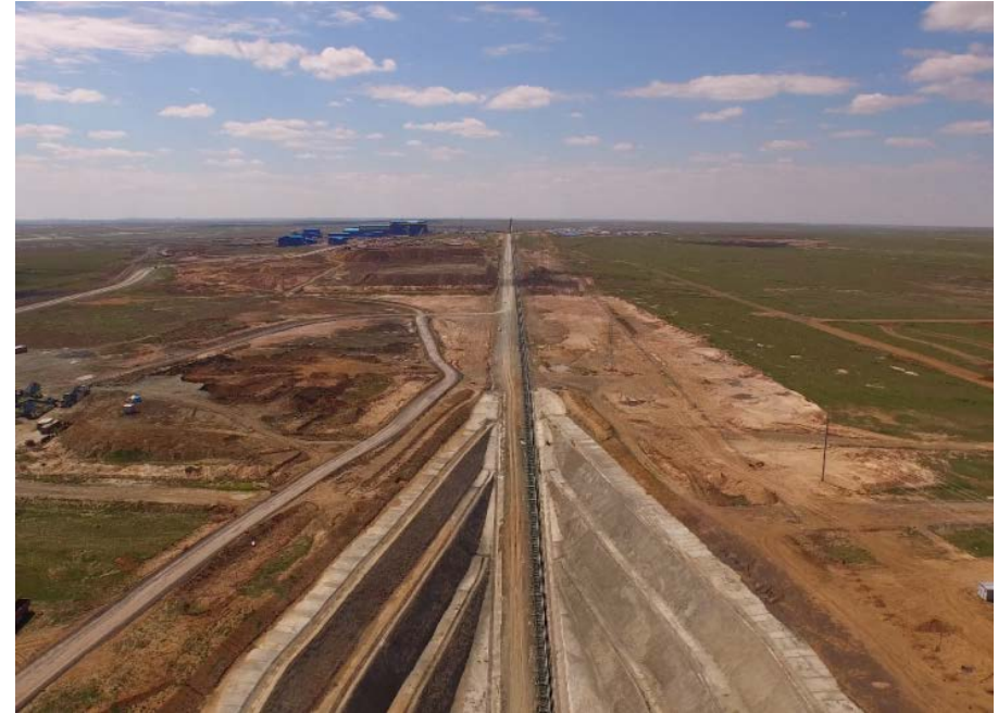
View from primary crusher
