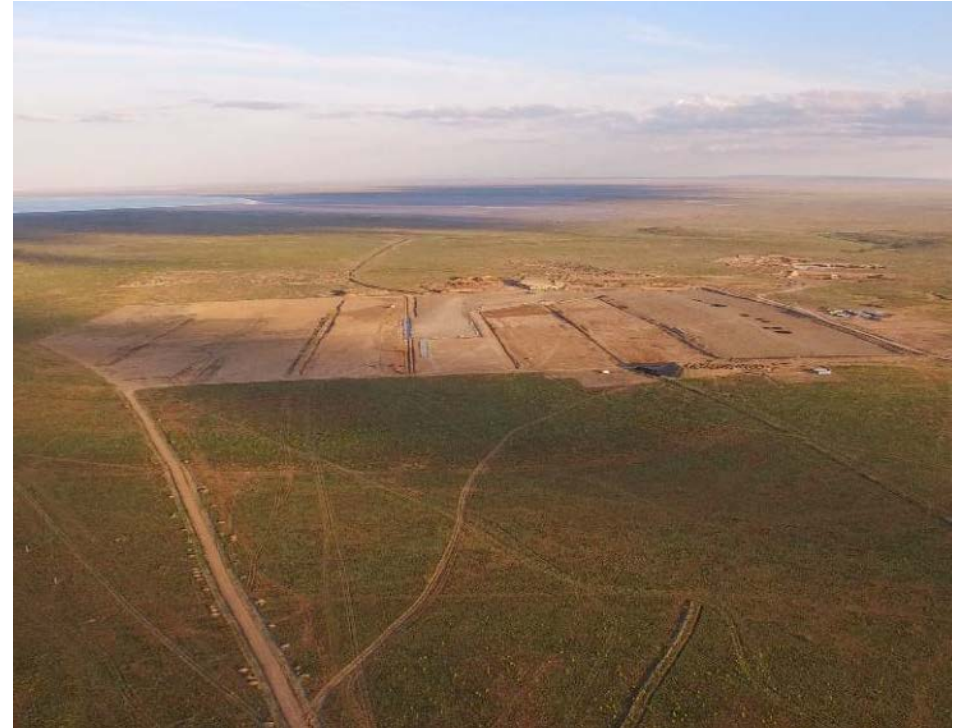
Heap leach cells 101-109 (right to left)
