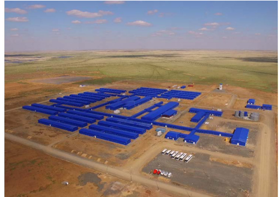
Permanent camp buildings
