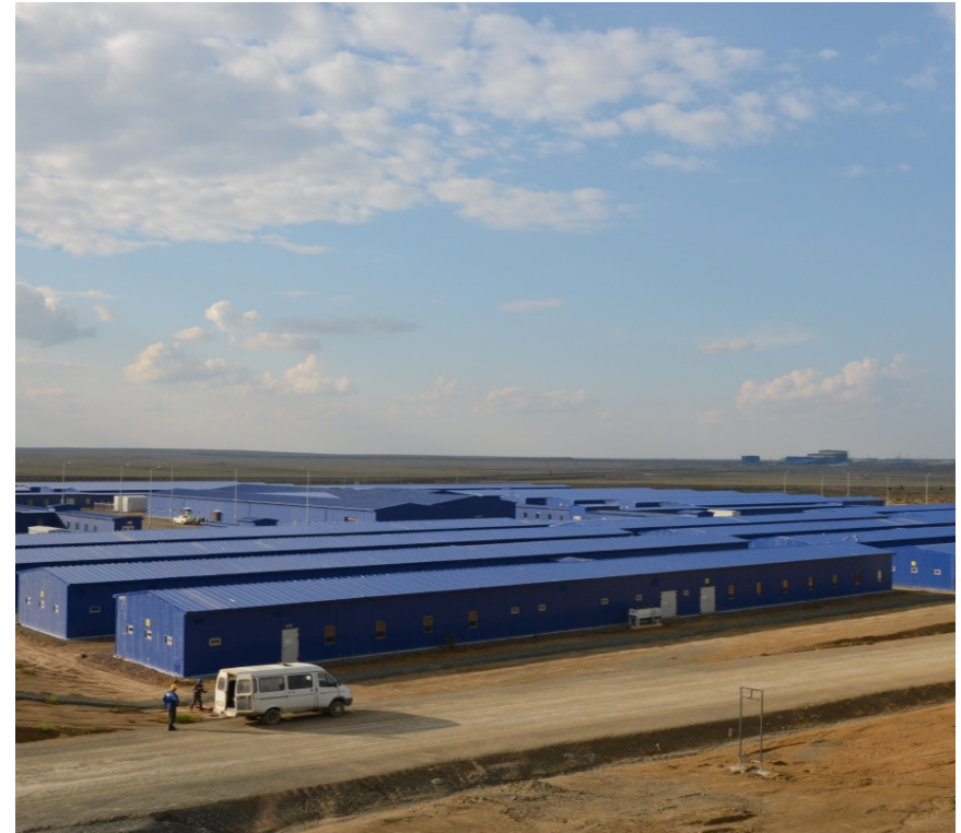
Permanent camp buildings
