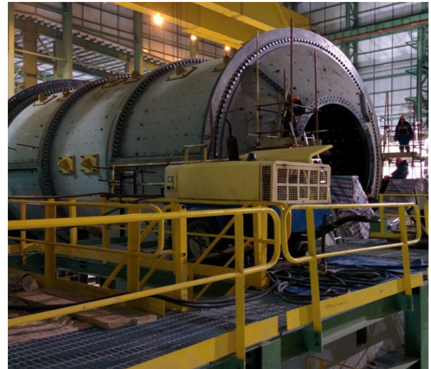
Ball mill mechanical installation
