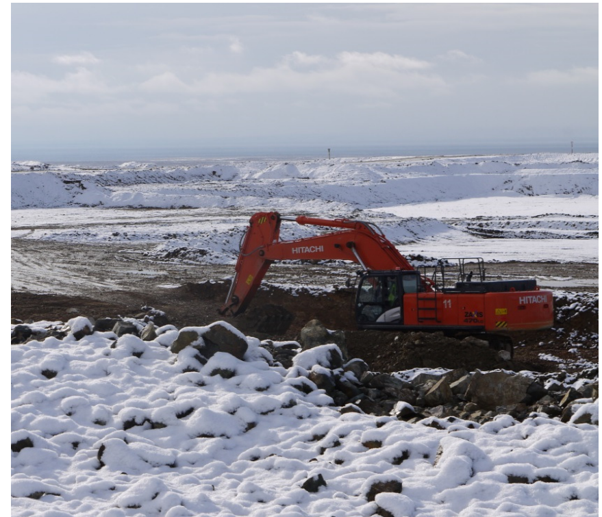
Sulphide concentrator bulk earthworks
