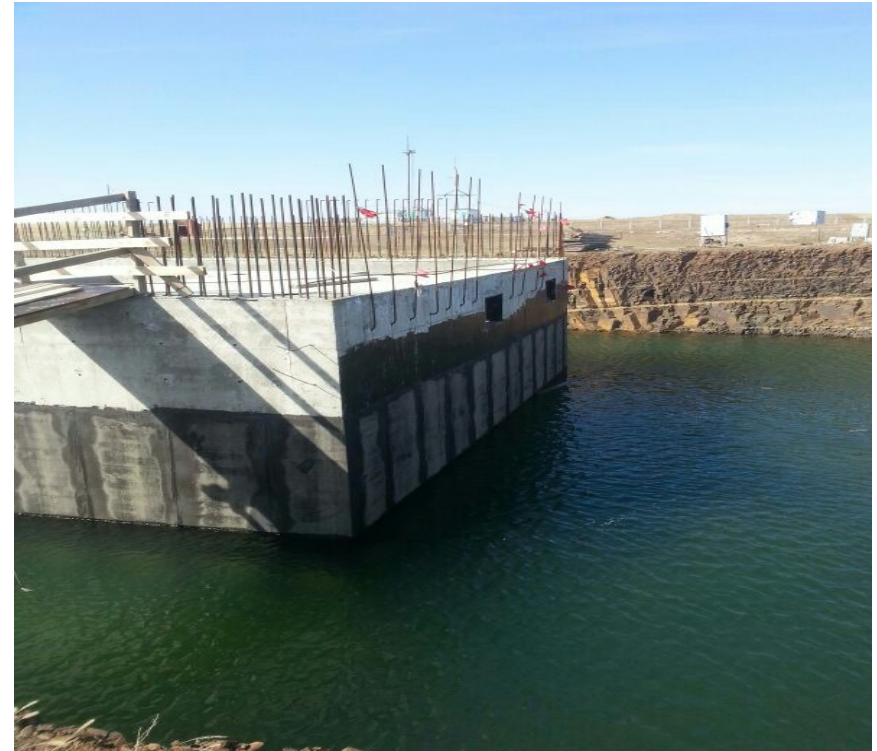
Water intake structure
