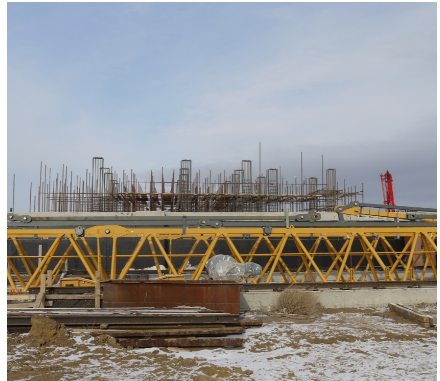
Clay plant steel work
