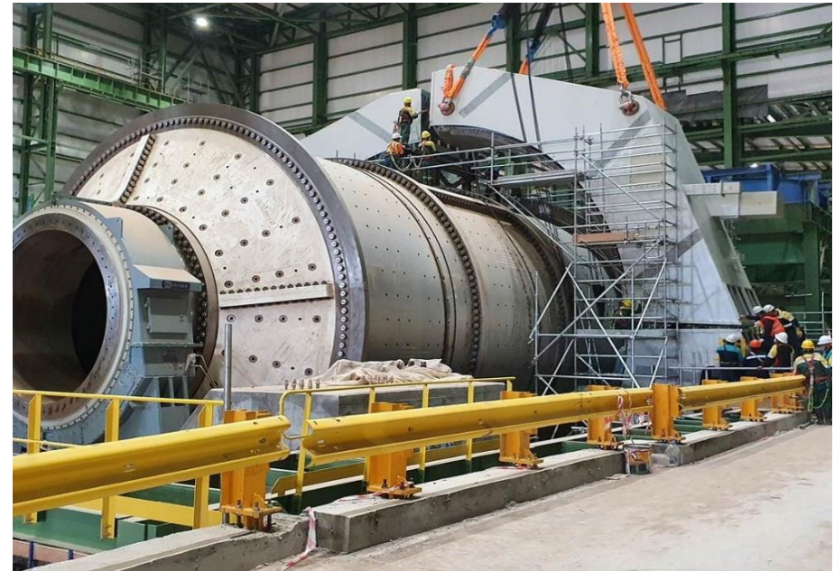
Ball mill 1 GMD installation, August 2020
