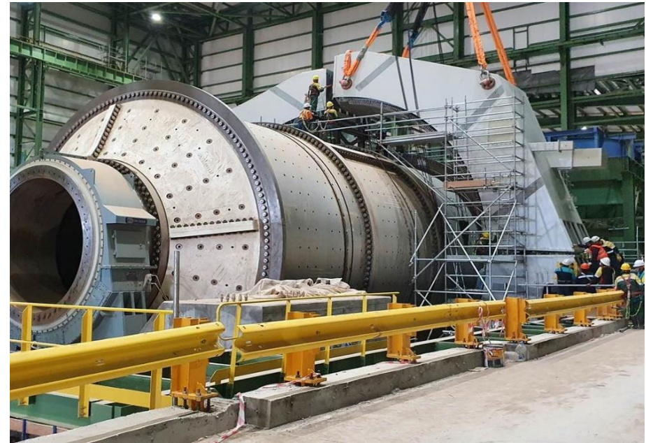
Ball mill 1 GMD installation, August 2020
