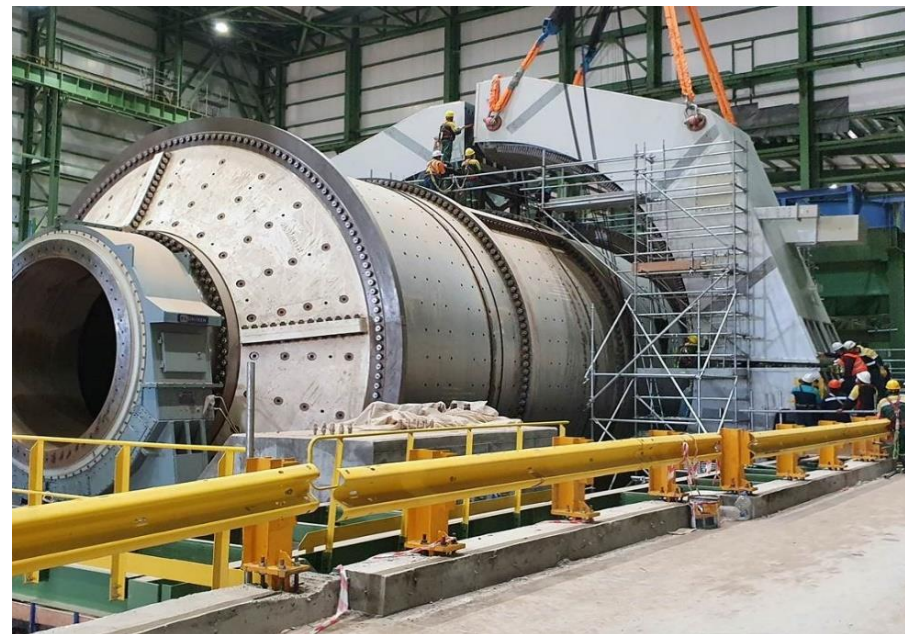
Ball mill 1 GMD installation, August 2020
