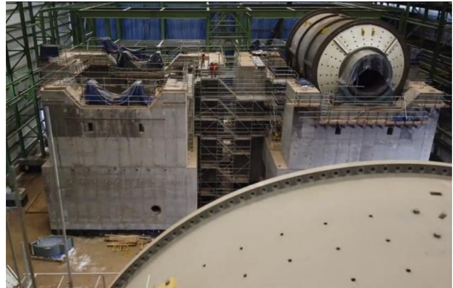
Mill installation works, January 2020
