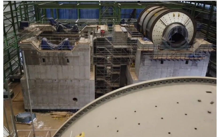
Mill installation works, January 2020
