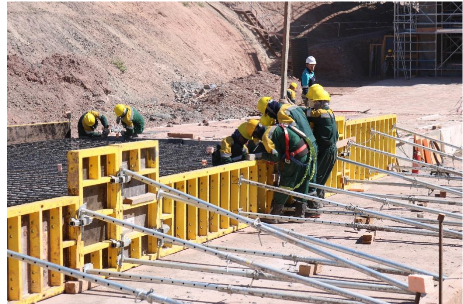
Aktogay II construction, June 2019
