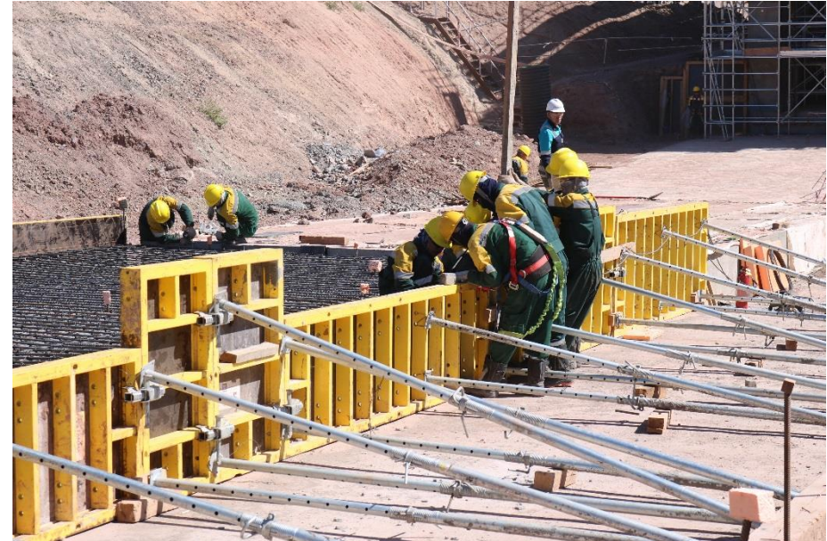
Aktogay II construction, June 2019
