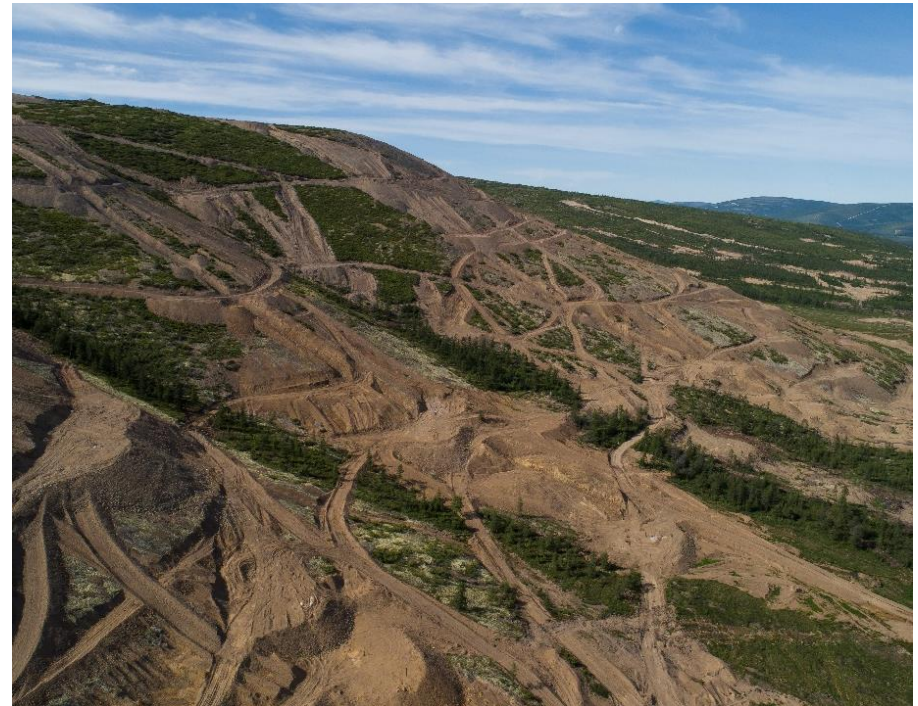
Peschanka deposit, Baimskaya copper project
