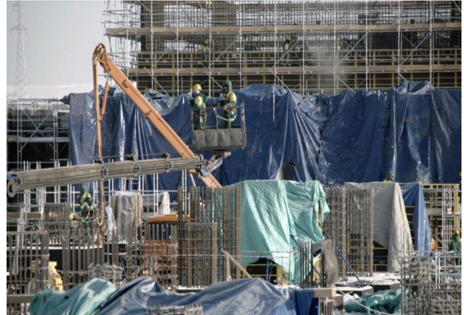
Structural steel works, Aktogay
