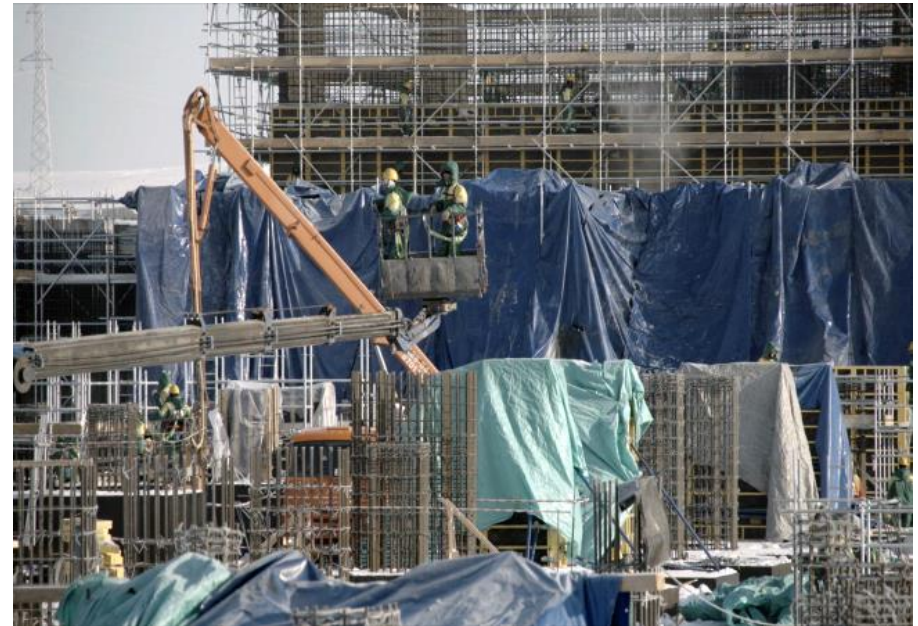
Structural steel works, Aktogay
