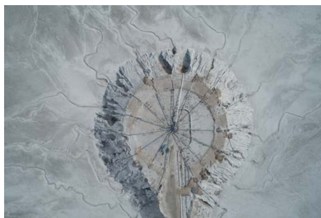
Aktogay tailings storage facility
